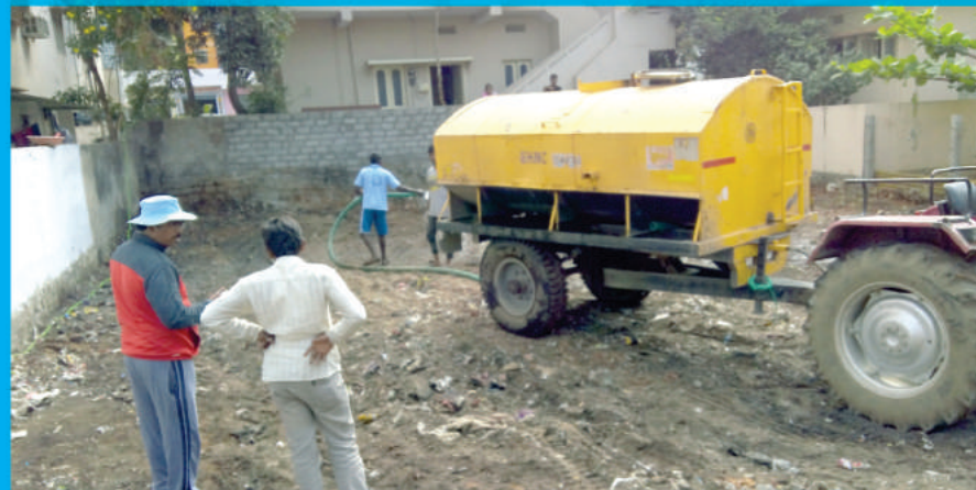
Spraying Water and filling up the area with several lorries of Mud
