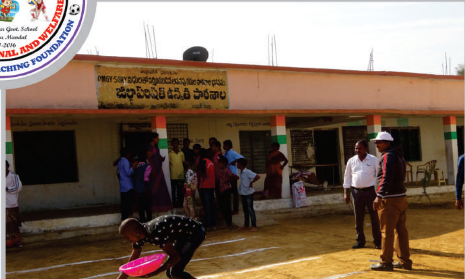
Ground Marking in progress...
