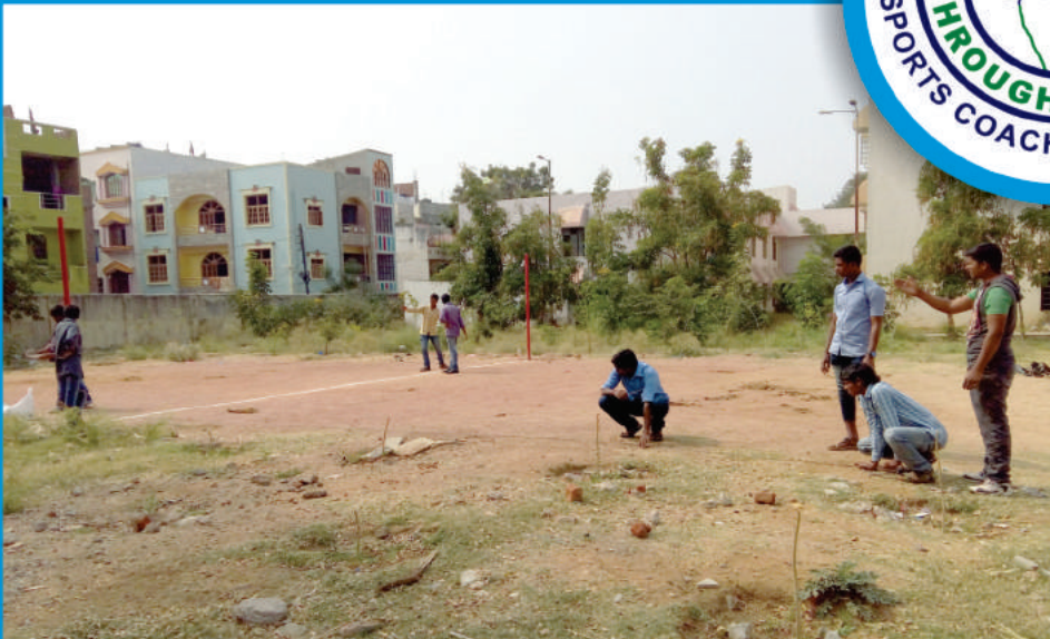
The appearance of the facility before!
